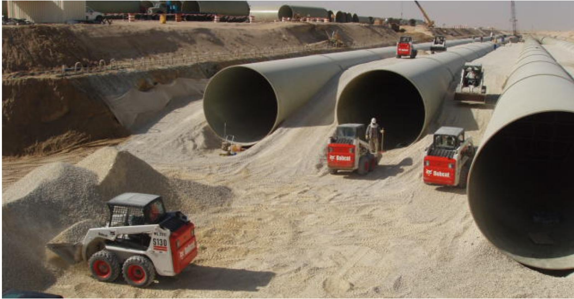
Figure 2.5: Very large FRP pipe systems from Future Pipe Industries ( www.futurepipe.com )
