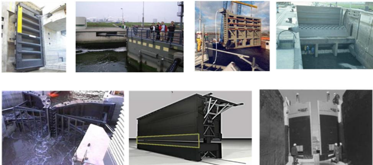
Figure 9.8: Different types of gates with innovative design/solution: (top L to R)- i) folded plate mitre gate (Uelzen, Germany), ii) reverse mitre gate (Ijmuiden-NL), iii) suspended mitre gate (NL), and iv) rotary segment (horizontal axis) lock gate (Lisdorf lock, Germany); (bottom L to R)- v) vertical axis sector gate, vi) lifting and sliding lock gate, and vii) Golbey composite mitre gate (Source: PIANC Workshop, Oct. 2009 presentations and other publications by same Working Group).
