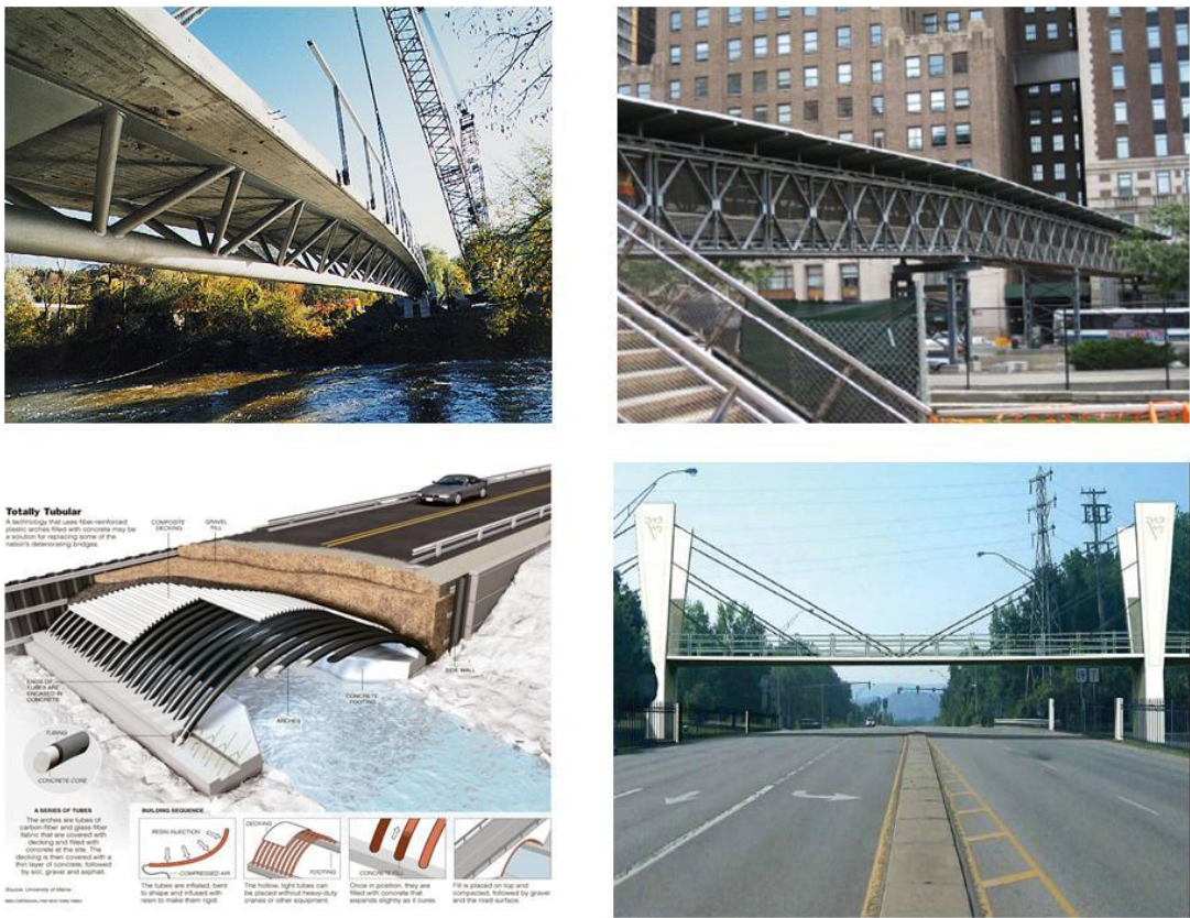
Figure 2.16: Examples of FRP application for bridges: (Top L to R)- i) Carbon cables used in bottom chord, Kleine Emme Bridge, Switzerland (Courtesy: Dr. Urs Meier); ii) FRP pedestrian bridge over 9 th Street, NY; (bottom L to R)- iii) Neal Bridge, Maine with FRP tubes (courtesy: NYTimes.com); iv) Proposed FRP Pedestrian Bridge at West Virginia University, Morgantown)
