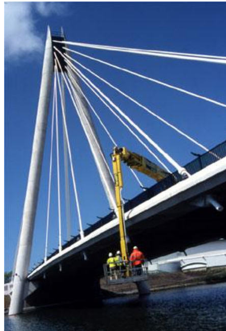
Figure 8.5: Bridge inspection using truck mount bucket, ( www.facelift.co.uk )
