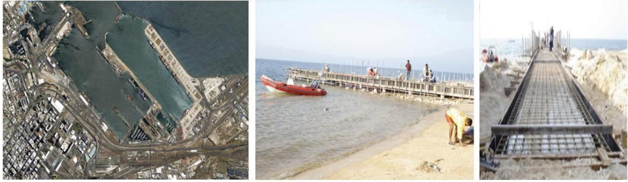
Figure 9.7: (L to R)- (i) Ben Schoeman Quay with FRP reinforced deck (2008), ii) GFRP reinforced concrete pier, iii) GFRP reinforcement for the concrete pier (top view) (Source: PIANC RecCom WG Report 105, 2009)
