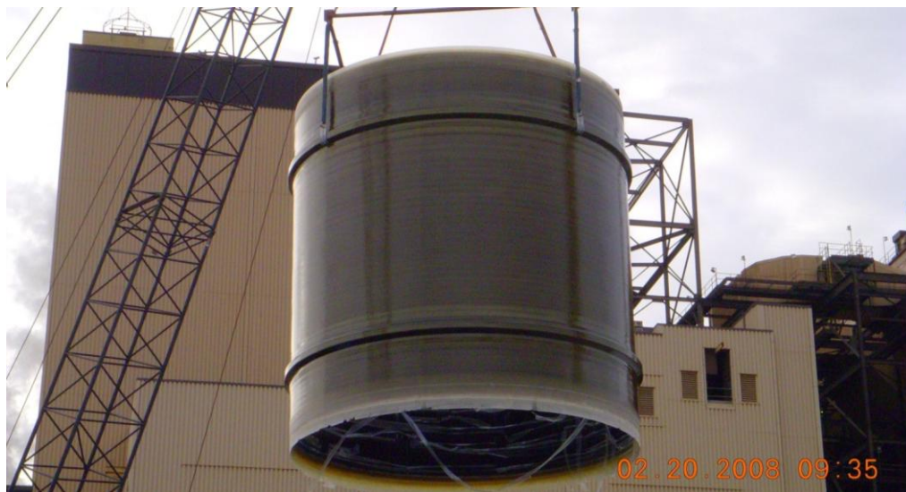
Figure 6.4: FRP composite chimney liner fabricated in field-plant through filament winding and used for smoke stack in a coal power plant, Morgantown, WV (Courtesy: CFC-WVU)
