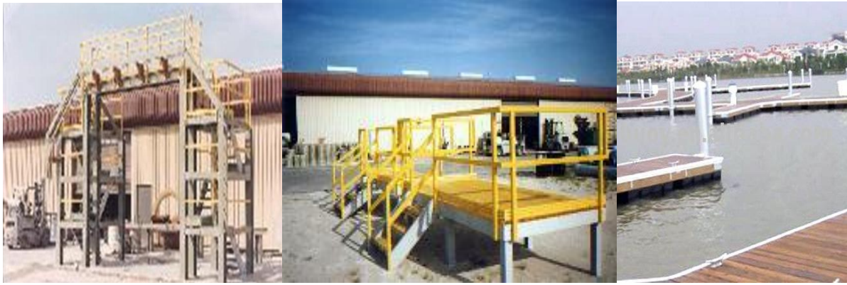
Figure 2.9: FRP Ground and Floating Platforms (Industrial Plastic Systems, Inc.)
