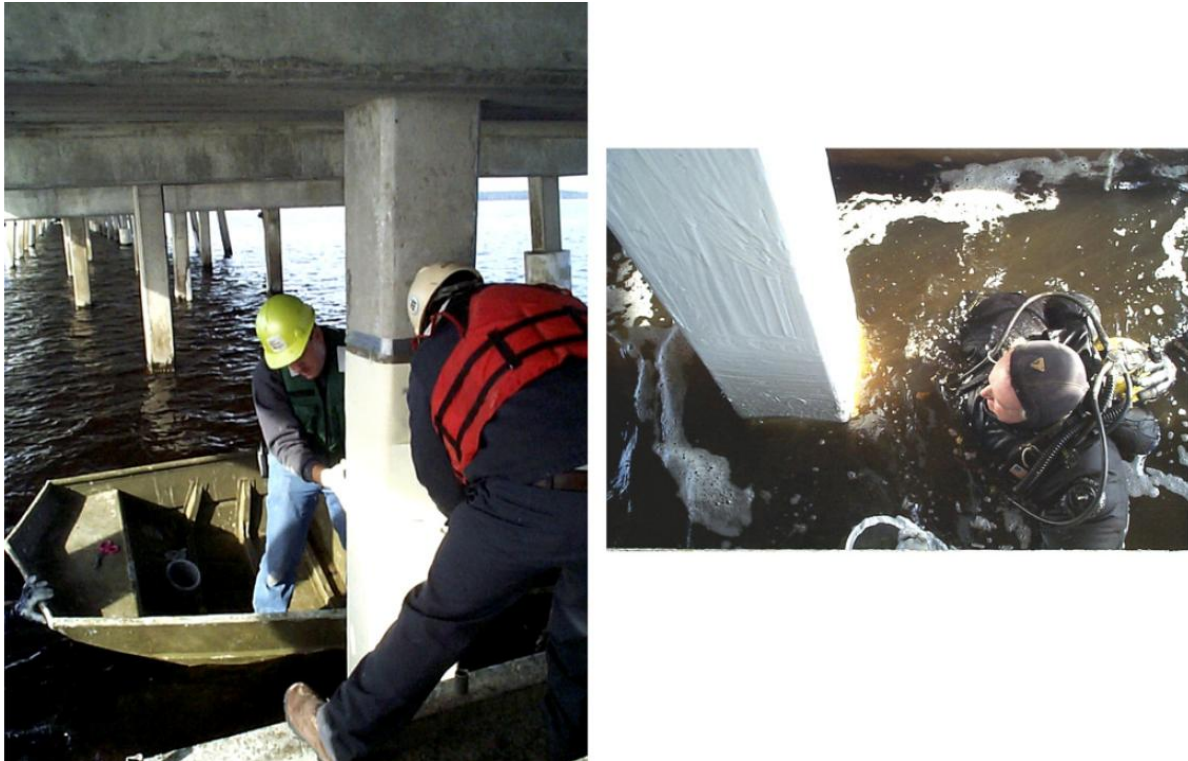
Figure 8.2: Underwater repair using a boat and divers (Courtesy Air Logistics), R. Sen and G. Mullins, 2007
