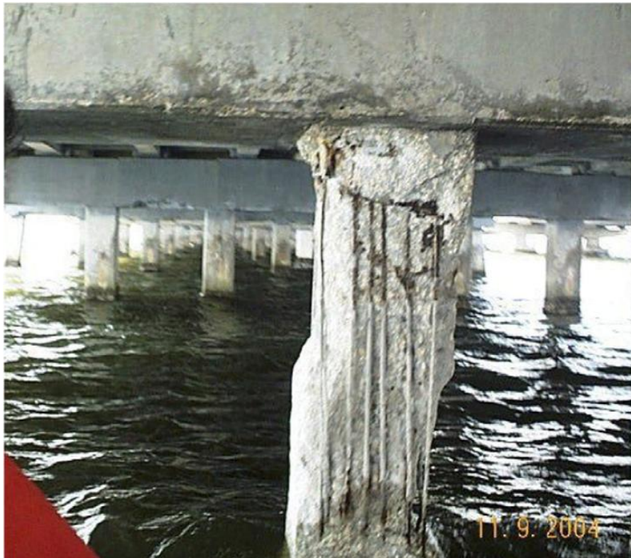
Figure 8.1: Damage to pile requiring emergency repair (Courtesy FDOT), Sen and Mullins, 2007
