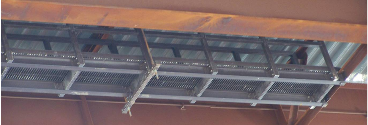
Figure 2.15 FRP Inspection Walkway Blennerhassett Bridge, Parkersburg, WV (Courtesy: CFC-WVU)
