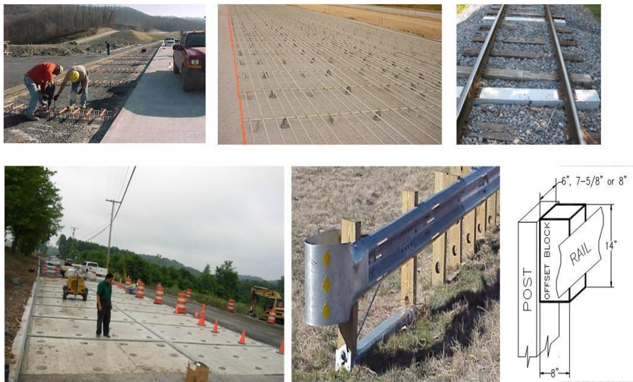
Fig. 2.12 : FRP Design and Applications by the CFC-WVU, (Top L to R) – i) FRP dowels in highway pavement (Elkins, WV), ii) FRP reinforcement for concrete highway pavement (Charleston, WV), and iii) FRP thermoplastic tie for railroads (Moorefield, WV); (bottom L to R) - i) FRP pavement panels (Morgantown, WV, iii) thermoplastic FRP offset block for guardrails, (Morgantown, WV) (Courtesy: CFC-WVU).
