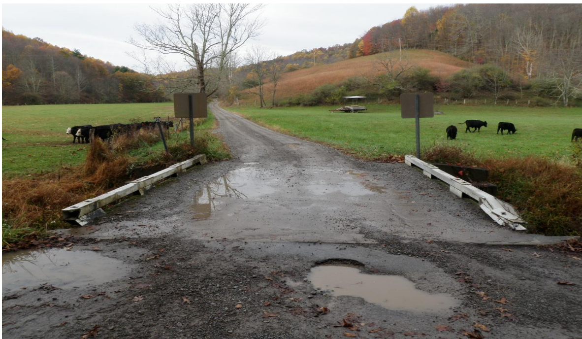
Fig. 8.10 FRP box section guardrail on a WV farm bridge (crushed under truck load on right) in need of guardrail replacement
