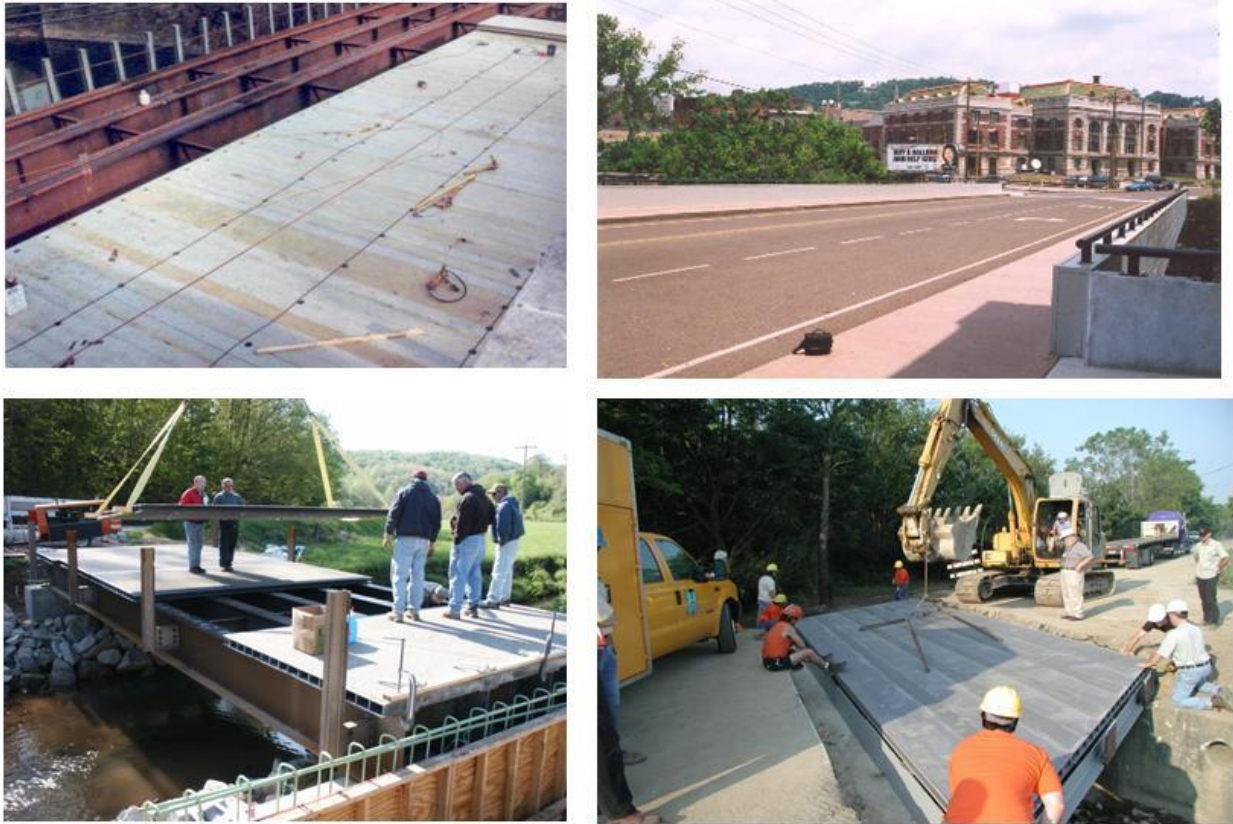
Fig. 2.13: FRP bridge deck shapes designed and field implemented in WV and Ohio by the CFC-WVU (Courtesy: CFC-WVU)
