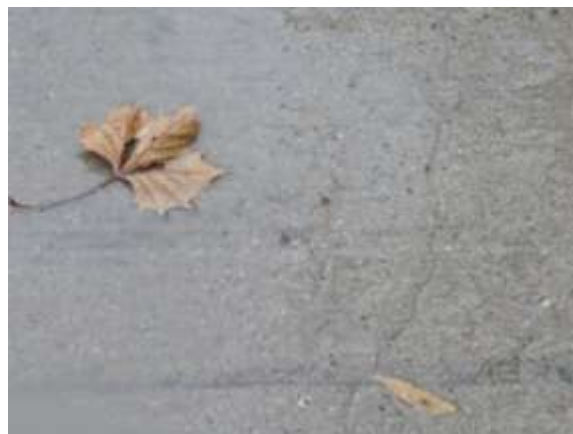
CRACKING IN DECK
