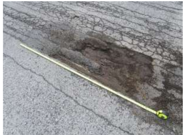
MISSING ASPHALT AT ABUTMENT 2
