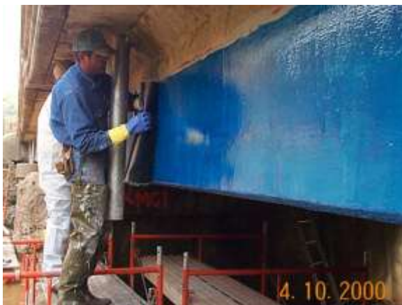
CFRP WRAP INSTALLATION
