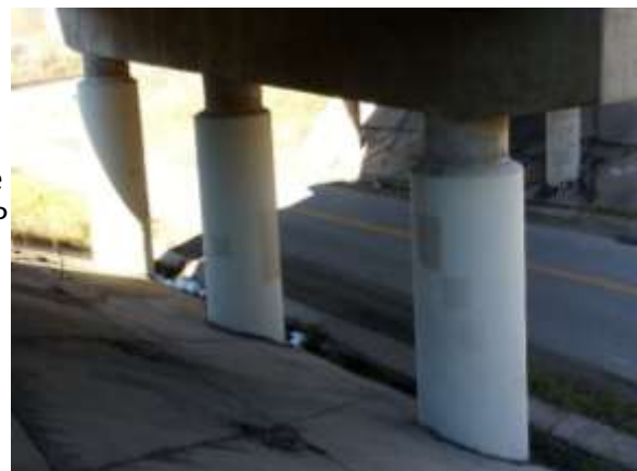
COLUMNS WRAPPED WITH FRP
