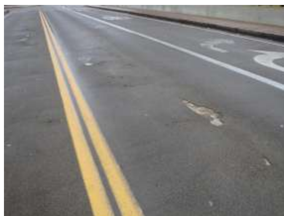
DELAMINATIONS IN WEARING SURFACE
