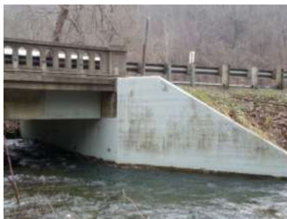
FRP WRAP ON WINGWALL AND T-BEAM
