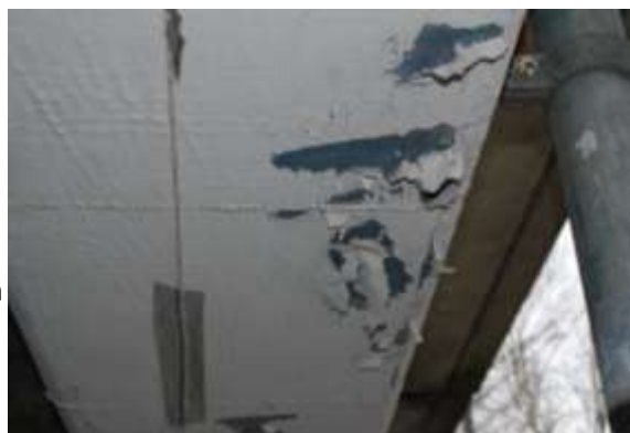
FAILED EPOXY COATING
