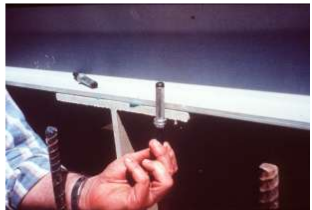
GALVANIZED STEEL BLIND BOLT (POP RIVET)
