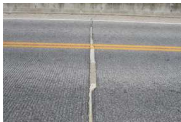
BREAKUP OF DECK PANEL JOINT
