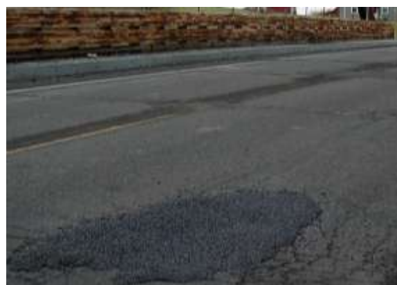
PATCHES IN WEARING SURFACE DUE TO FRP DECK FAILURE
