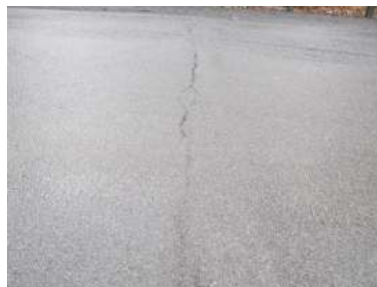
TYPICAL TRANSVERSE CRACKING
