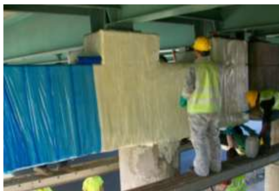
INSTALLATION OF THE FRP WRAP
