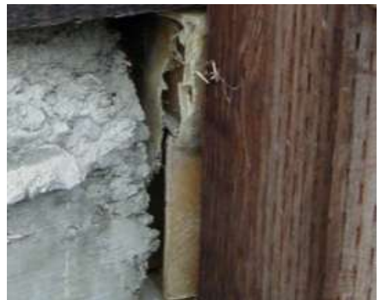
LOCALIZED FAILURE OF FRP DECK
