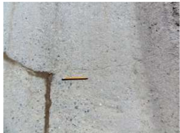
HAIRLINE CRACKS IN DECK
