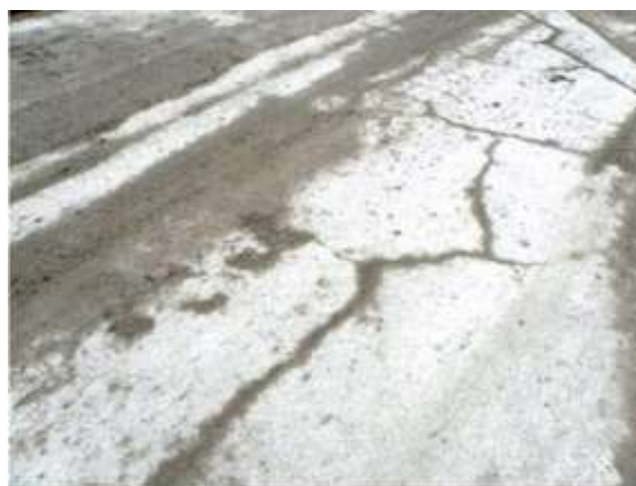
MAP CRACKING IN DECK
