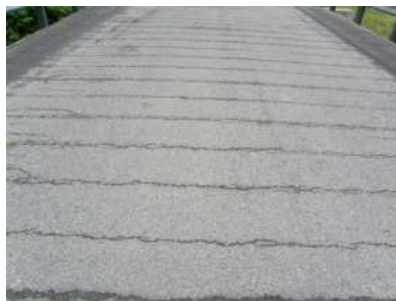
TRANSVERSE CRACKS IN WEARING SURFACE
