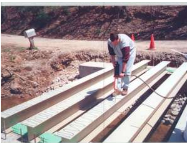
APPLICATION OF PLIOGRIP ADHESIVE TO GFRP BEAMS
