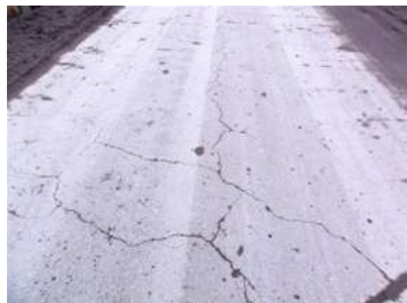
DECK CRACKING
