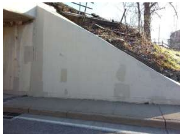
WINGWALL REPAIRED WITH FRP WRAPS
