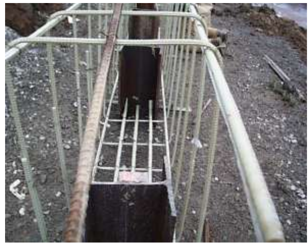
CLOSE UP OF REBAR IN ABUTMENT
