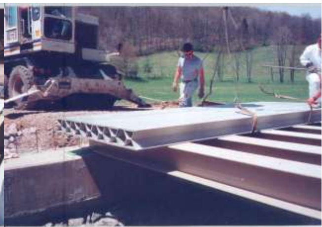
INSTALLATION OF DECK PANELS
