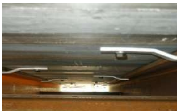
Z-CLIPS ATTACHING DECK TO BEAMS
