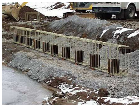
GFRP REINFORCEMENT IN ABUTMENTS
