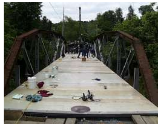
DECK PRIOR TO WEARING SURFACE INSTALLATION
