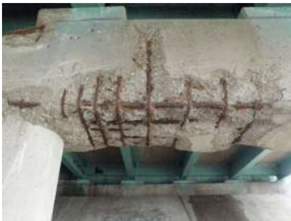
CONCRETE DETERIORATION PRIOR TO REPAIR
