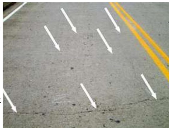
CRACKS IN THE WEARING SURFACE
