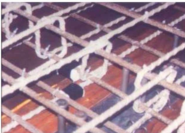
GFRP REINFORCEMENT IN DECK WITH STEEL SHEAR STUDS
