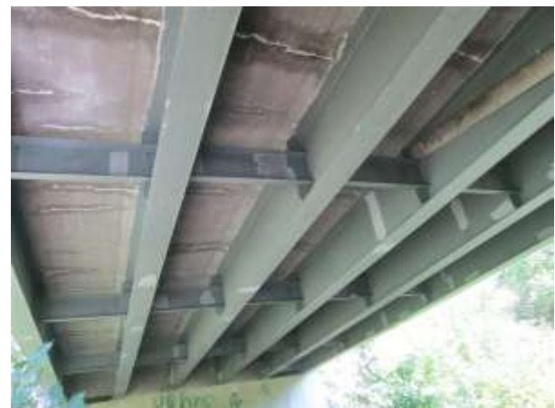
UNDERSIDE OF DECK WITH CRACKS/EFFLORESCENCE
