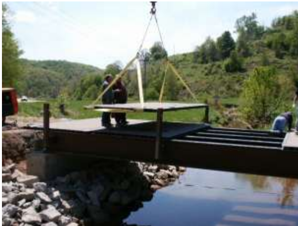
PLACEMENT OF DECK PANEL
