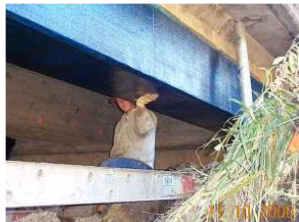
BLUE EPOXY WRAP PRIOR TO PAINTING
