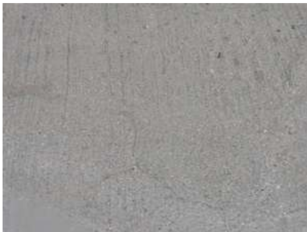
MAP CRACKING IN DECK
