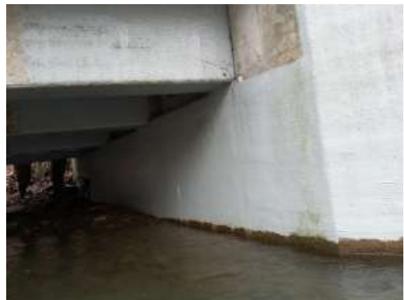
FRP ON T-BEAM, ABUTMENT AND WINGWALL
