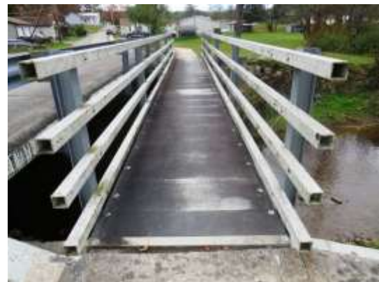
FRP SIDEWALK ADJACENT TO BRIDGE
