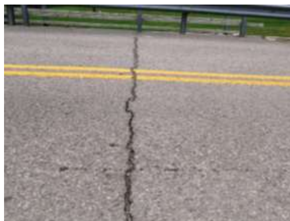
WEARING SURFACE CRACK
