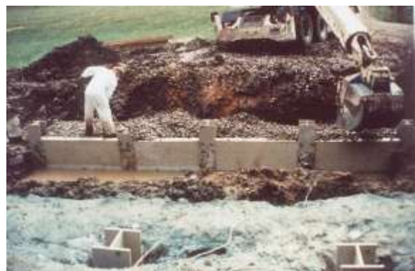
GFRP PILES/CELLULAR LAGGING MODULES
