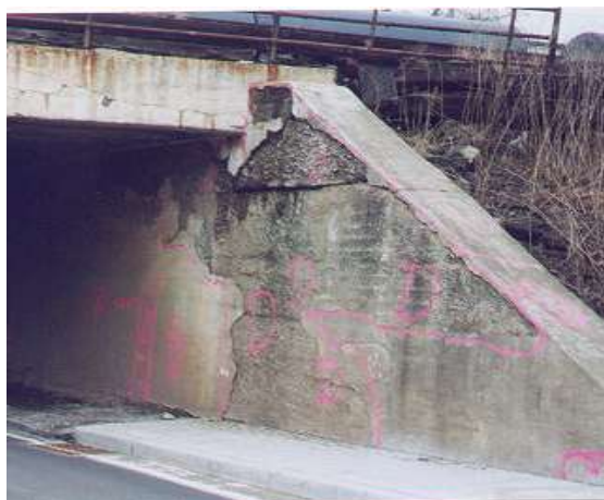
WINGWALL PRIOR TO REHABILITATION
